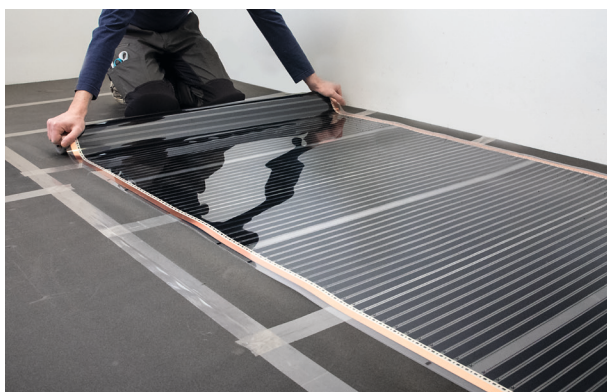
2 Installera QuickHeat systemet
